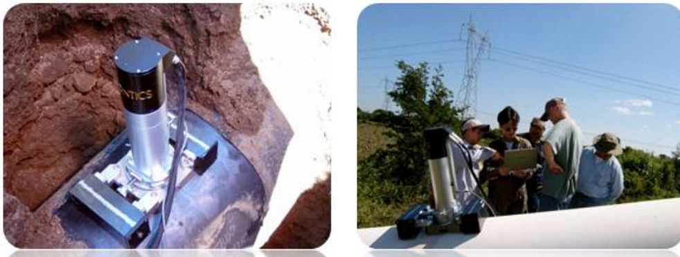
그림 20. Application cases for natural gas pipeline inspection using non-destructive indentation technique (PEMEX pipeline tests with GE PII members in Mexico)
